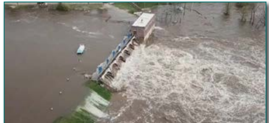
Sanford Dam Failure - Midland County (outside region)
